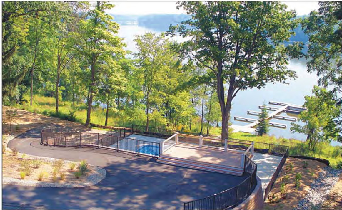
Some homes at Lake Chapin Shores in southwest Michigan have lakefront views, and some have lake and woods views, but all have access to the community's common areas, which include a heated pool, waterfront and private piers.
